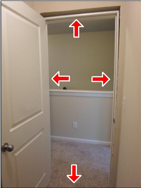
14.2 Item 3(Picture) missing weather stripping and threshold
