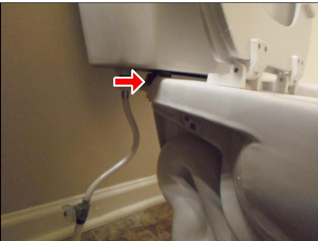
15.9 Item 1(Picture) leaking toilet
