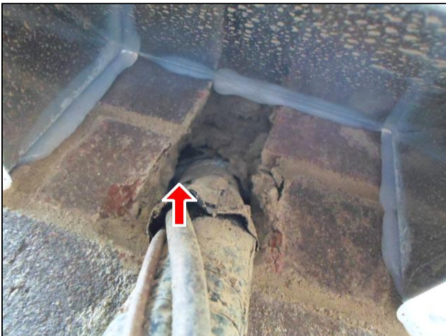
3.0 Item 3(Picture) ac line not sealed properly
