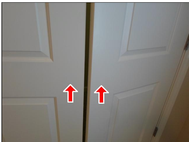
16.4 Item 1(Picture) missing door knobs
