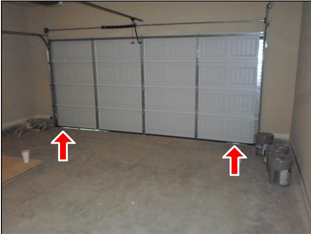
4.3 Item 1(Picture) gaps below door when closed
