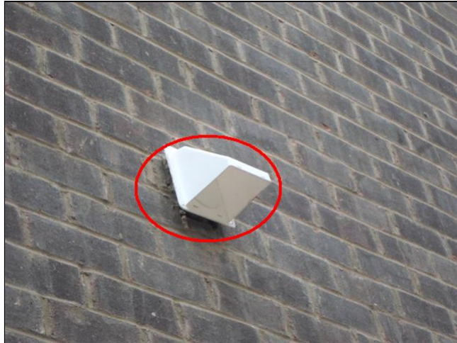
3.0 Item 2(Picture) vent not sealed properly
