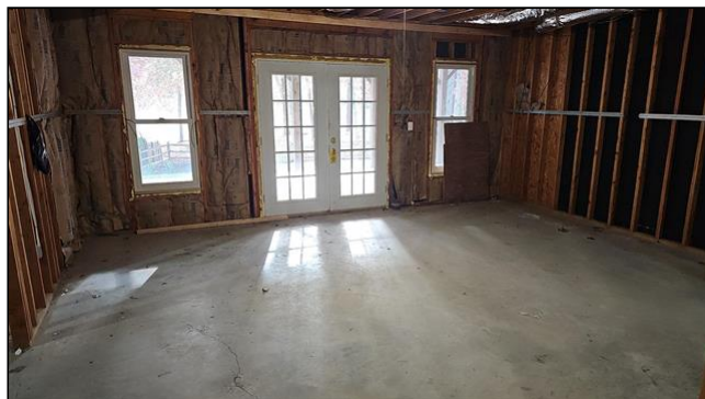
rear center basement room
