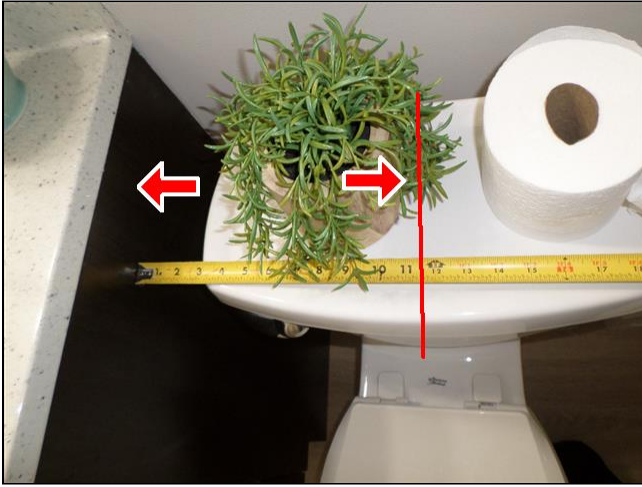
15.8.D Item 1(Picture) toilet near cabinet
