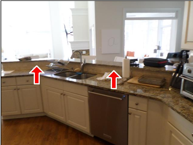
6.5 Item 1(Picture) missing outlets
