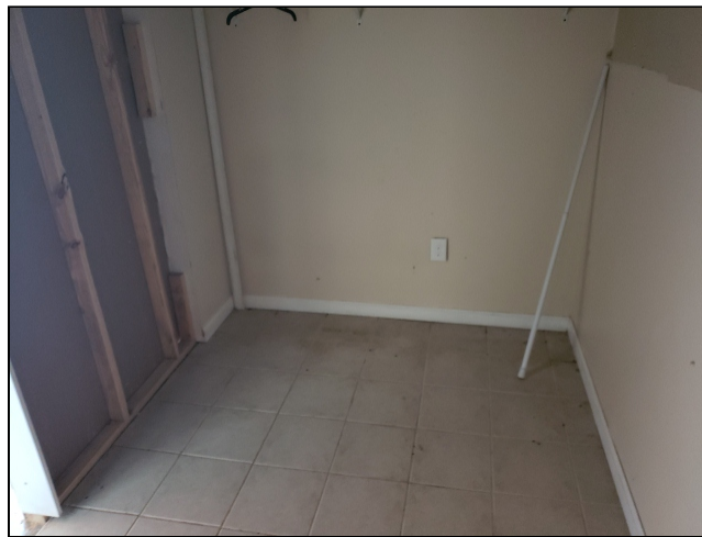
rear center basement room
