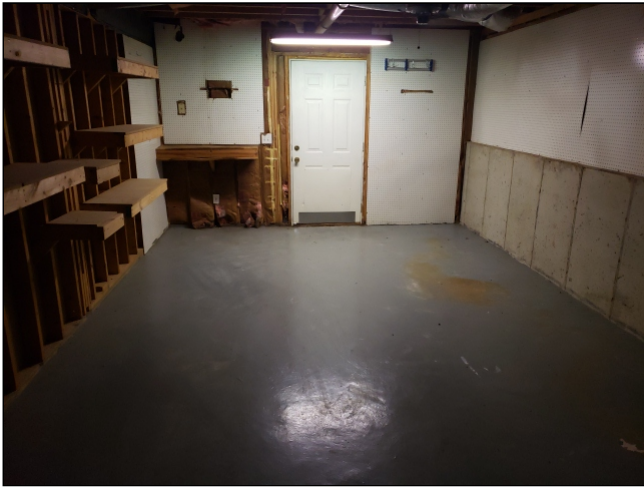
right basement room
