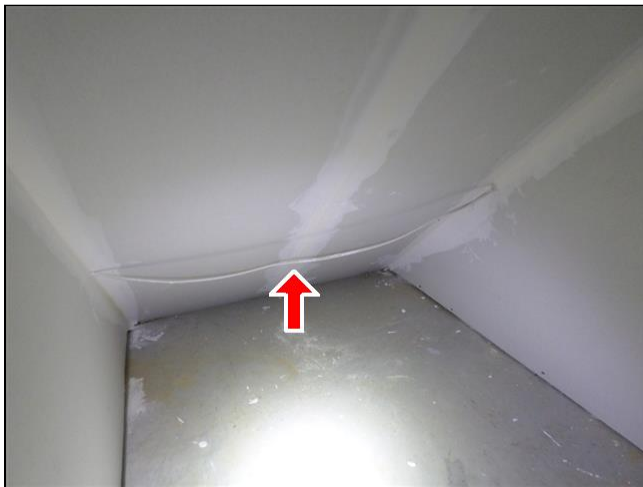
7.5 Item 1(Picture) loose wire
