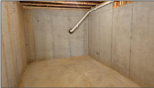
front left basement room
