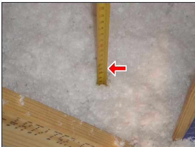
14.2.B Item 1(Picture) low insulation
