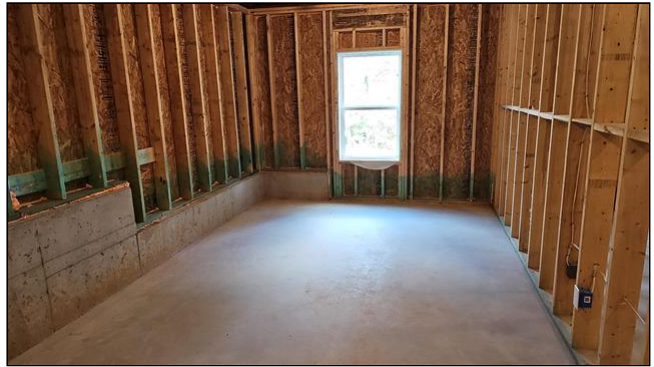
rear left basement room
