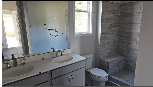
1st floor bathroom
