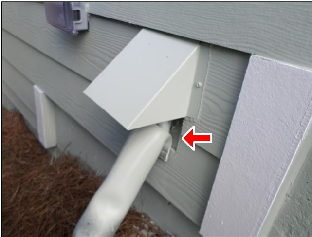
3.0 Item 2(Picture) exposed osb
