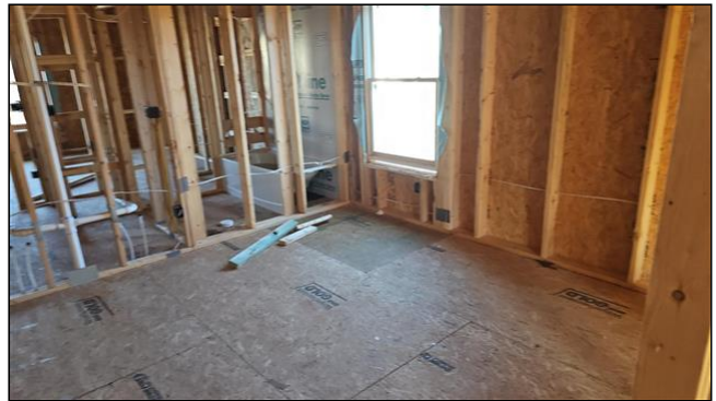
rear 2nd floor bedroom
