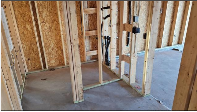
right 1st floor hallway
