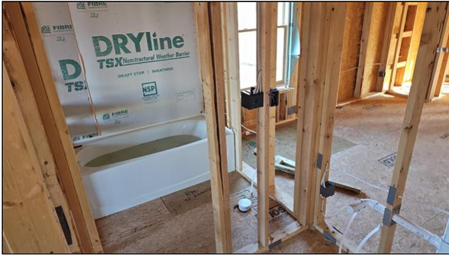
front 2nd floor bathroom
